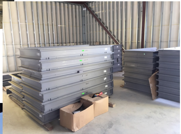
SW MS – Material Storage – H.M. Frames.
